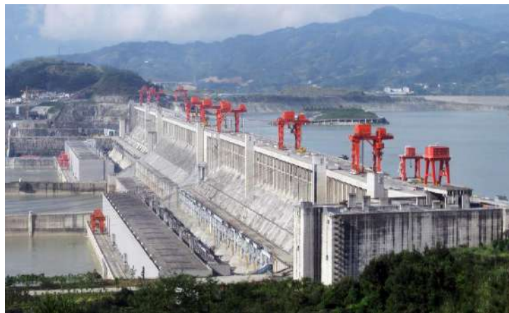
Figure 4 Hydroelectric power plants [12]
